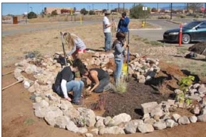
Fig. 1. MASTERS students stabilizing basin berms and spreading mulch.
