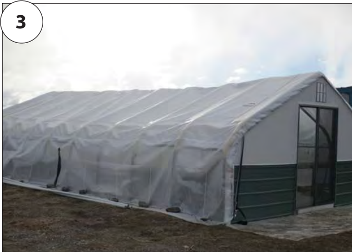
Notice the slit midway down the length. It allows us to roll up the bottom five feet of the cover for even more airflow, which will harden up our seedlings.
