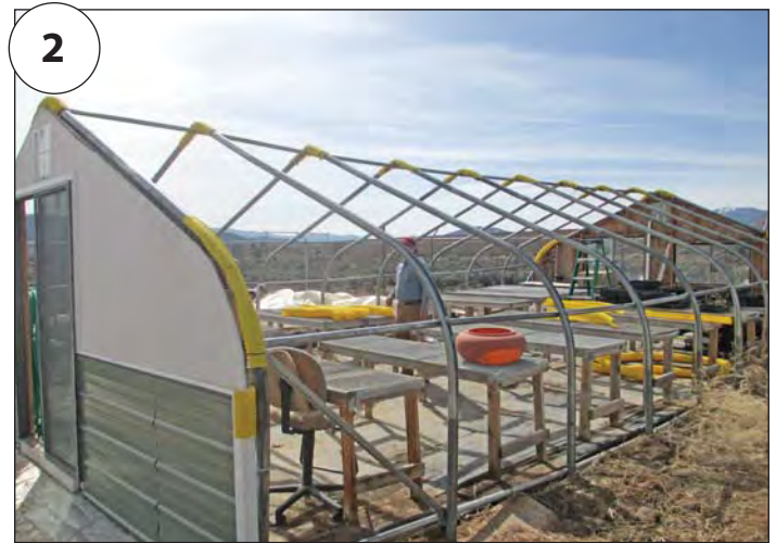
. . . cut some vents into the peak for even more airflow . . . wrapped the pipe frame of the greenhouse in yellow baseball fence tubing to keep it from rubbing.
